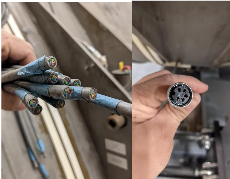
Fig.1. Strain gauge load sensor old cables (left picture) and connector already installed on magnet (right picture)
